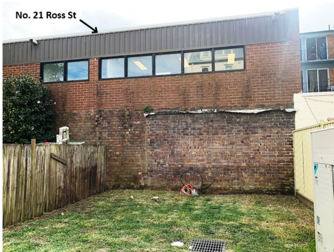
view to adjacent commercial building fronting Ross Street
